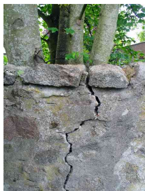
Figure 12g: Biological weathering by trees: roots opening up a crack in a rock and trunks pushing against a wall.
