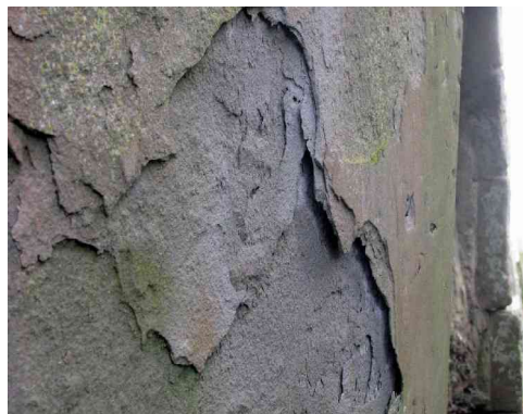
Figure 12b: Physical & chemical weathering of a gravestone
